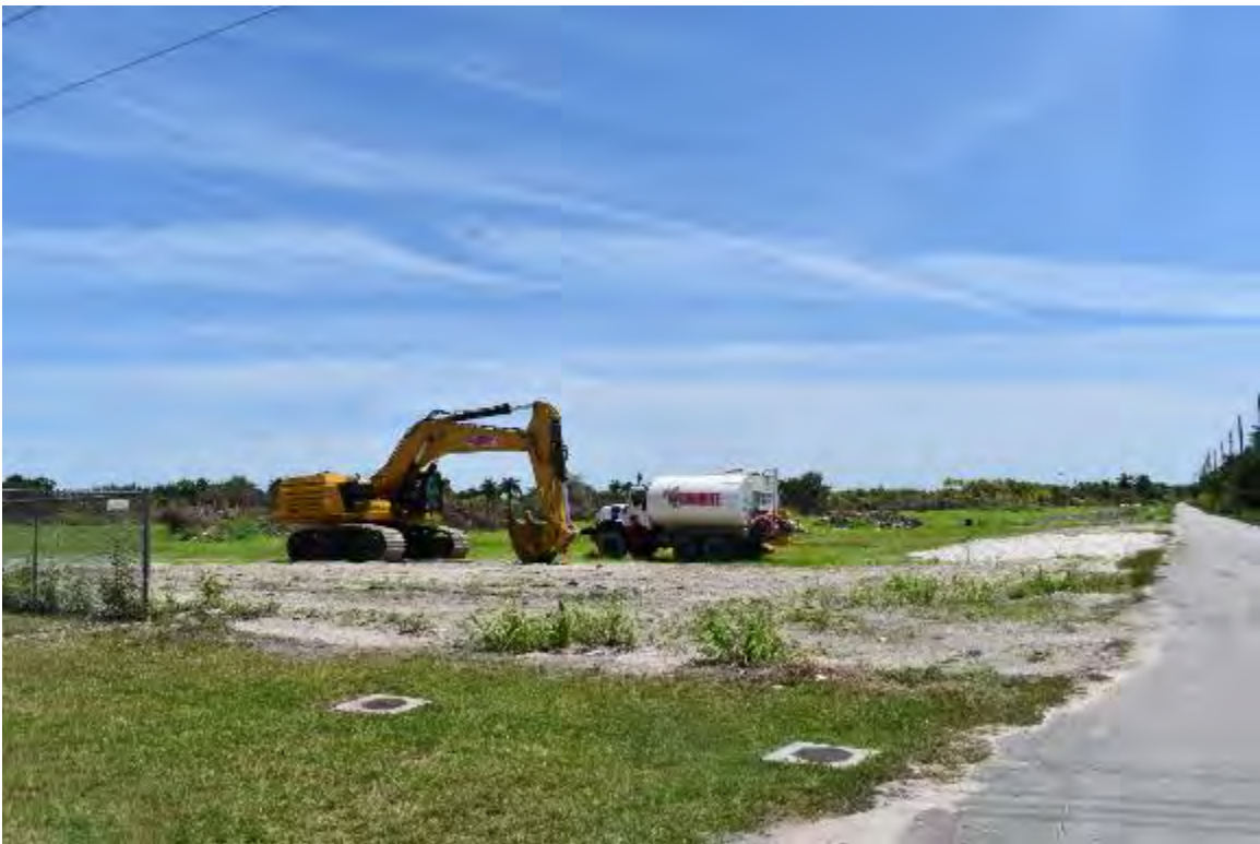
View looking southeasterly from northwest corner of property.
