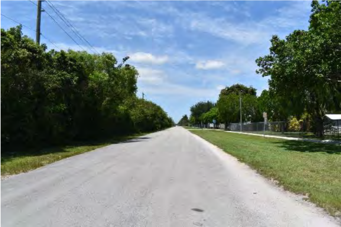
View looking northerly along SW 180 th Avenue.
